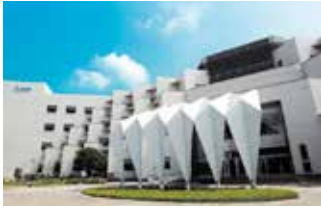
Tainan Plant (Diamond-rated Green Building)
