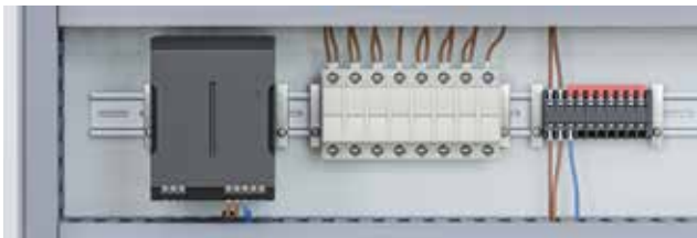
Wiring and short-circuit bars are required between devices
